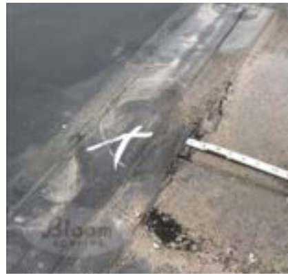
Failed field patch
