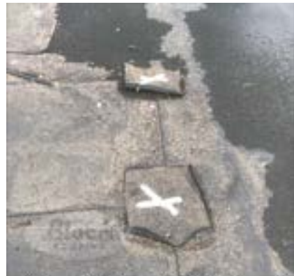
Failed field patch
