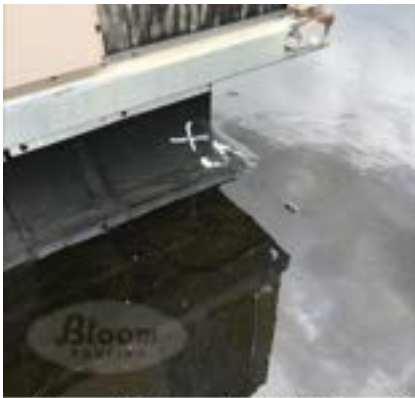
4 failing patches around this unit Roof is ponding 2" of water around this unit
