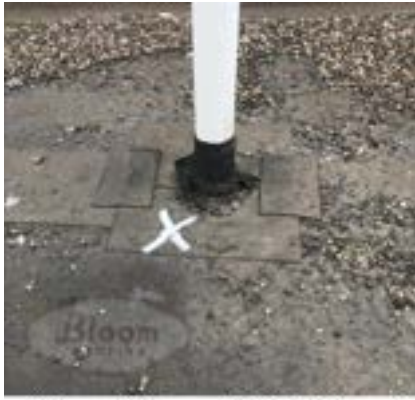
Failed pipe penetration flashing
