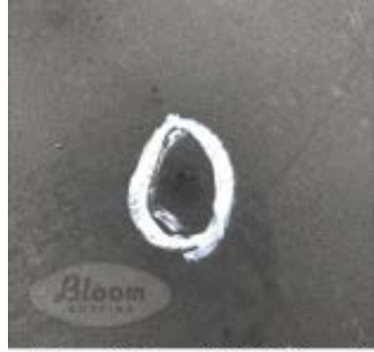
Hole in membrane
